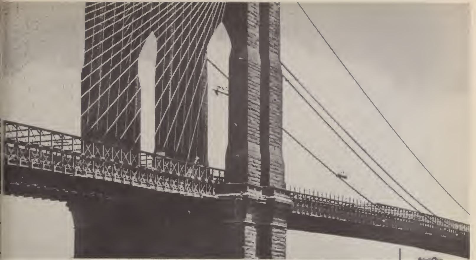
Brooklyn Bridge, before the heightened trusses along the outer edges were completed—note section immediately right of tower.
